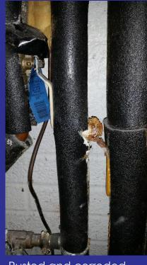
Rusted and corroded domestic water valve
